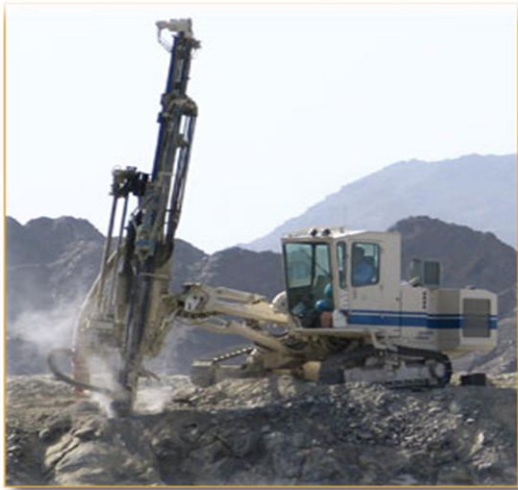
The pattern of drill holes being prepared for blasting.
